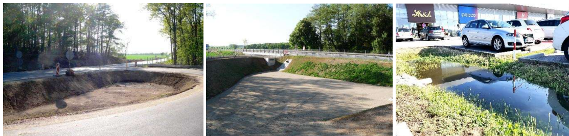
Collecting rainwater from transport infrastructure and parking lots in reservoirs (example from Austria)
