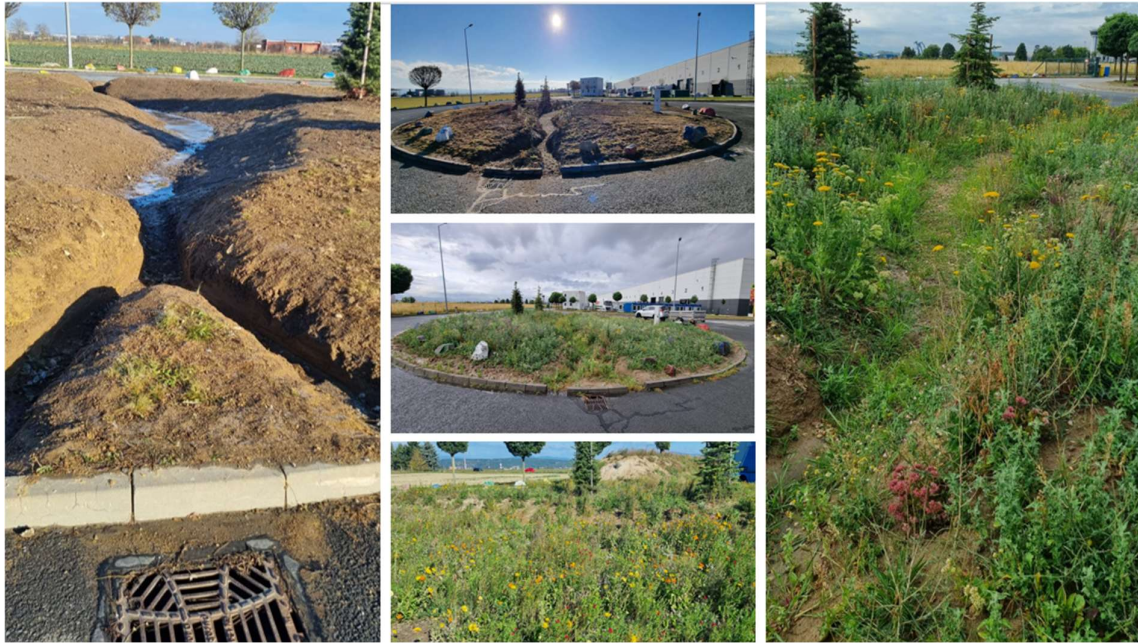
Rainwater from transport infrastructure was redirected into the centre of a roundabout (CTP industrial park, Košice)
