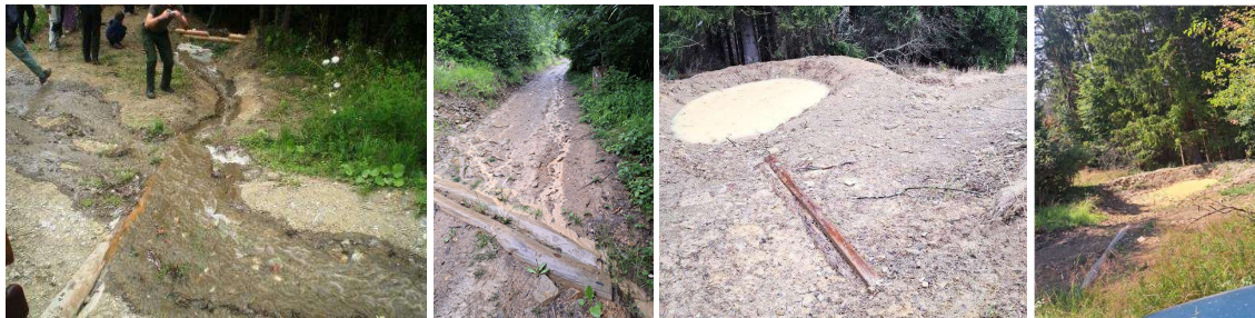
Water bars with infiltration pits
