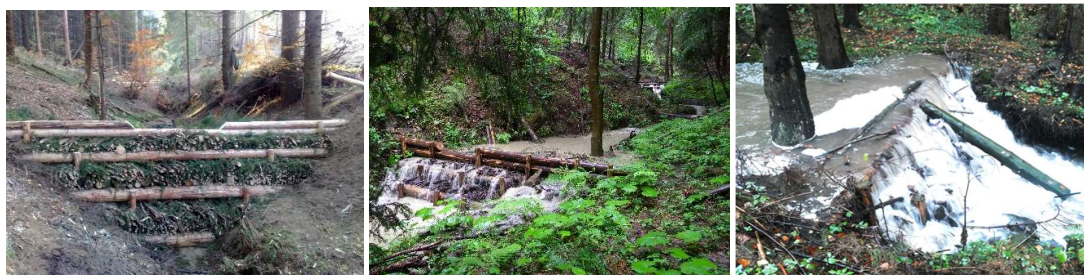
Impact of brushwood dams on the water regime of periodically drying small watercourses (Snežnica, Skalité, Oščadnica)
